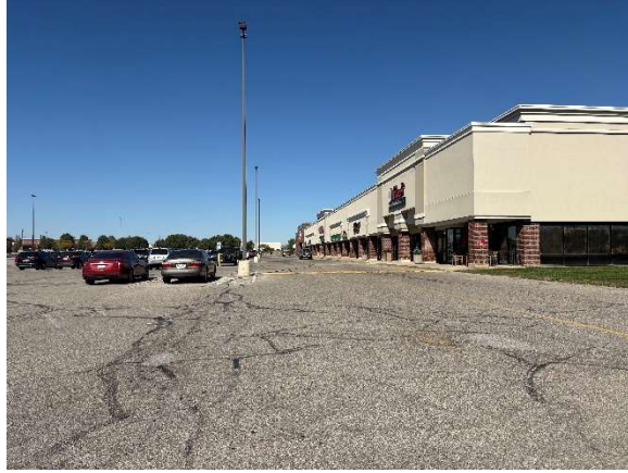
Kroger's (looking north)
